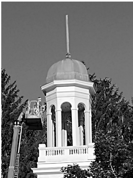
Scraping and painting of the cupola
