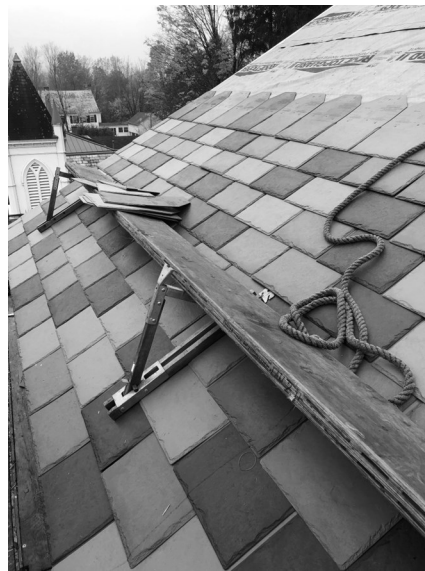
Town Hall roof synthetic slate installation
